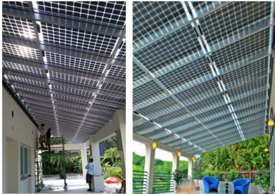
Figure 14. Shading Architectural Elements with Photovoltaic Panels
