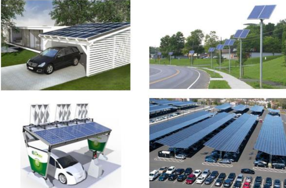
Figure 15. Parking Structures with Photovoltaic Panels that provide shading systems and also functional changing of electro-mobiles
