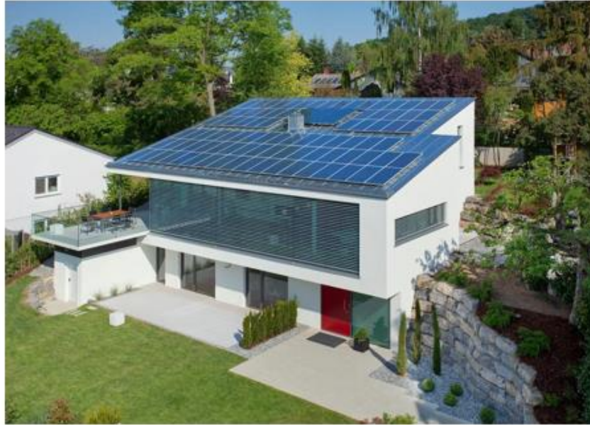
Figure 7. Roof with Photovoltaic Integrated Panels that follow the shape and angle of the roof system
