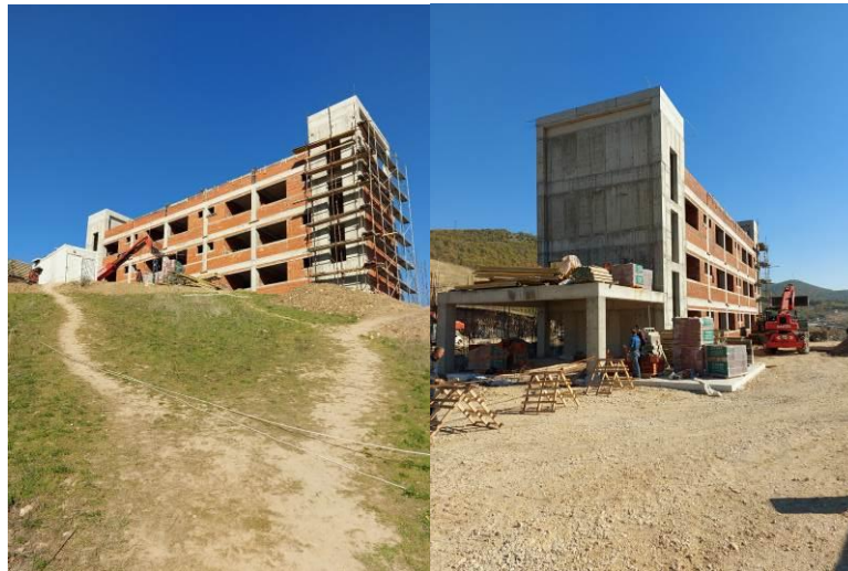
Figure 7. Photos of the construction site
