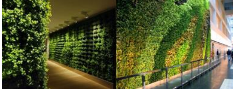
Figure 3. Living wall composed of individual planting cells on supporting panel system
