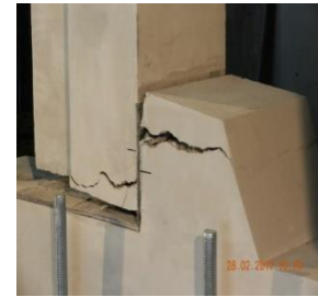
Fig. 12. Damage of M3-B improved connection
