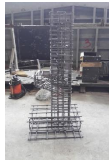
Fig. 5. Reinforcement of column with corbel
