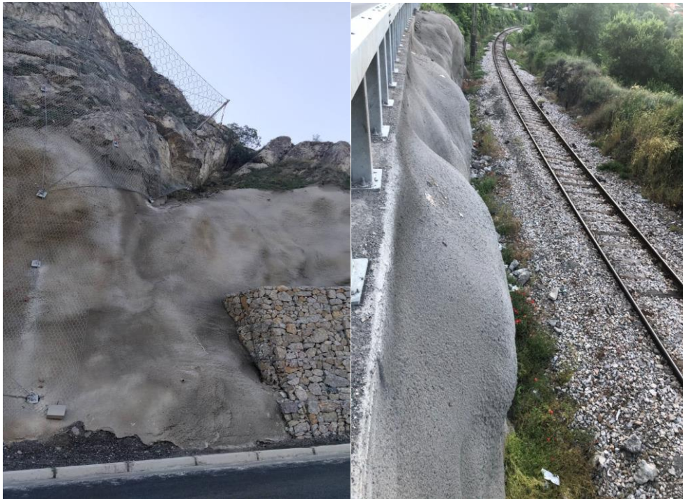
Figure 2. Construction of shotcrete on regional road R1102, section Veles - Gradsko
