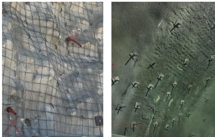
Figure 1. a) embedded mesh and b) embedded anchors
