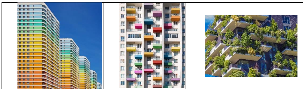
Figure 6 Design aesthetics of buildings facades using different colors and contract shapes and materials
