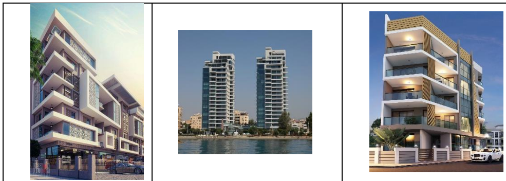
Figure 3 Aesthetics of international examples of Residential Buildings
