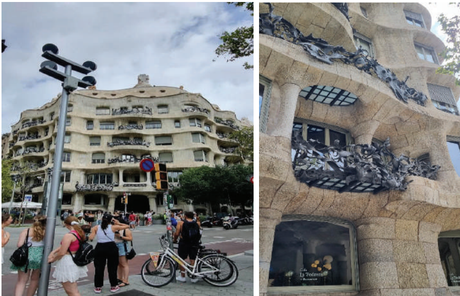
Figure 2 Antoni Gaudí's Casa Milà as an example of biomimicry in architecture [private photos]
