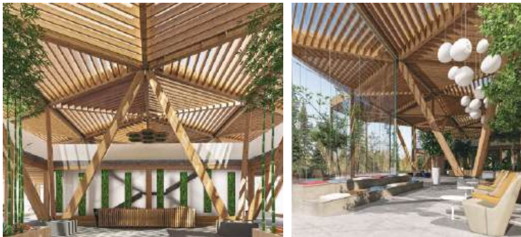
Figure 7 Project proposal for a Botanical Garden in Skopje with a structural system from GLT, designed by Faton Kalisi, master student at the International Balkan University
