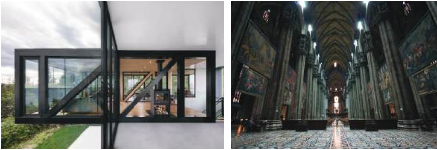
Figure 4 a) Milan Cathedral in Milan, Italy, where the vaults are displayed and are adding an aesthetic quality to the building ( https://traveldigg.com/milan-cathedral-du-omo-di-milano/ ); b) A truss house by ACDF* architecture in La Malbaie, Canada, with exposed steel truss ( https://architizer.com/blog/inspiration/collections/truss-houses/ )
